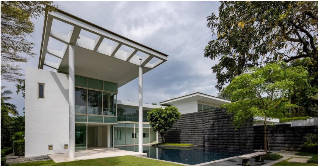
The exterior of the GCB in the neighbourhood of Belmont Road designed by Mok Wei Wei sits on a prime freehold site of 15,898 sq ft (Photo: Samuel Isaac Chua/EdgeProp Singapore)
